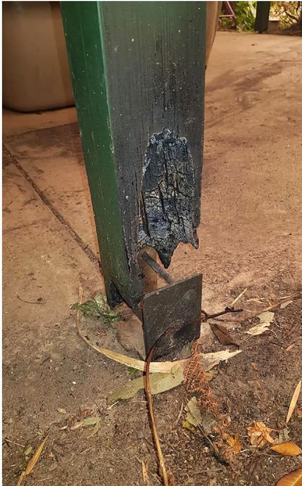
Figure 6. Structural timber elements can quickly become a fire conduit into the main home (Image: Nadia Edwards by permission of Author).
