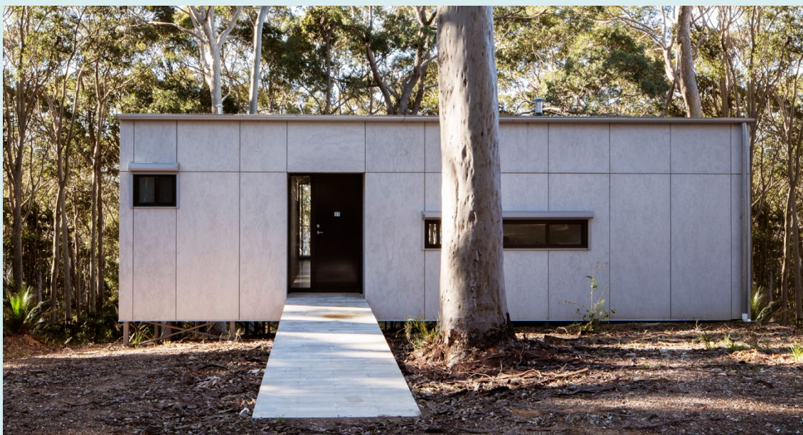
Figure 3. A simple form and non-combustible materials are two of the key defensive features of this house (Image: Ross Caddaye).
