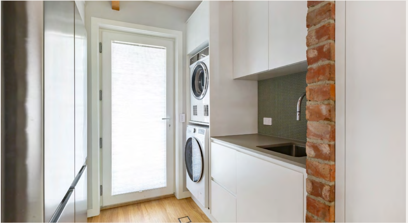
↑ Provide somewhere inside where it's easy to fill buckets, and a readily accessible tap to connect a hose for interior fire defence. This laundry has a washing machine tap in the cupboard under the sink. Image: Ben King
